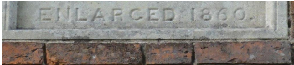
Picture 3: When was this building erected and what is its name?
